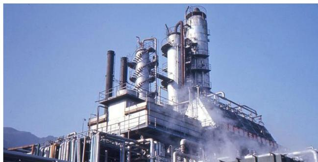
The plants are part of an experimental project and will employ toluene and hydrogen to exploit the hydrodealkylation reaction, yielding benzene.
